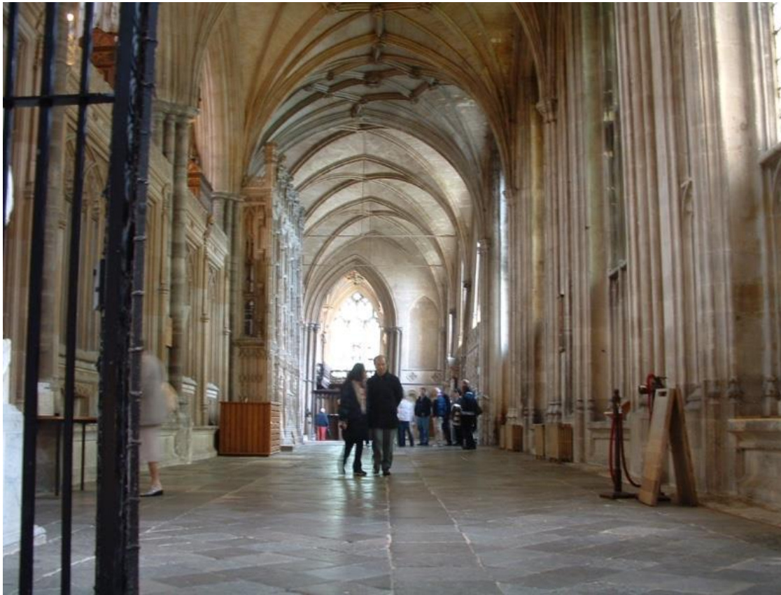
Winchester Cathedral south wall (right side) bowing out. Notice the rods across the aisle just below the arches. (My photo)
